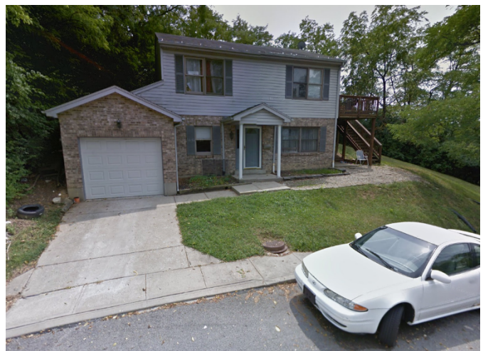
Figure 1. Original house before fire damage
